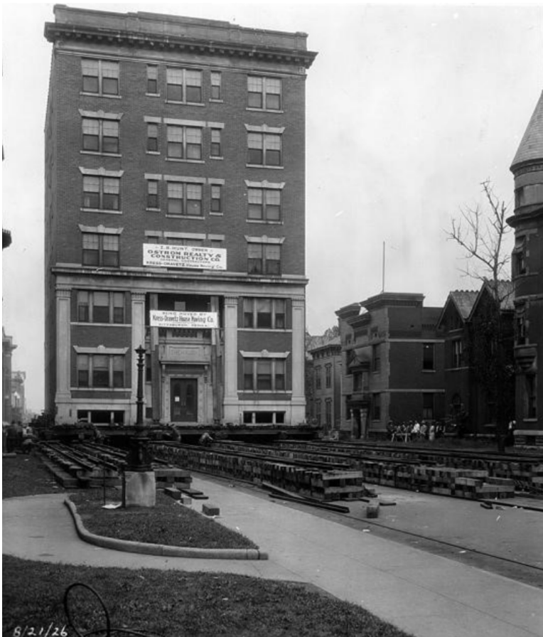
Moving Haugh Hotel from site on Michigan Street out of path of War Memorial Building, 1926. War Memorials Commission
