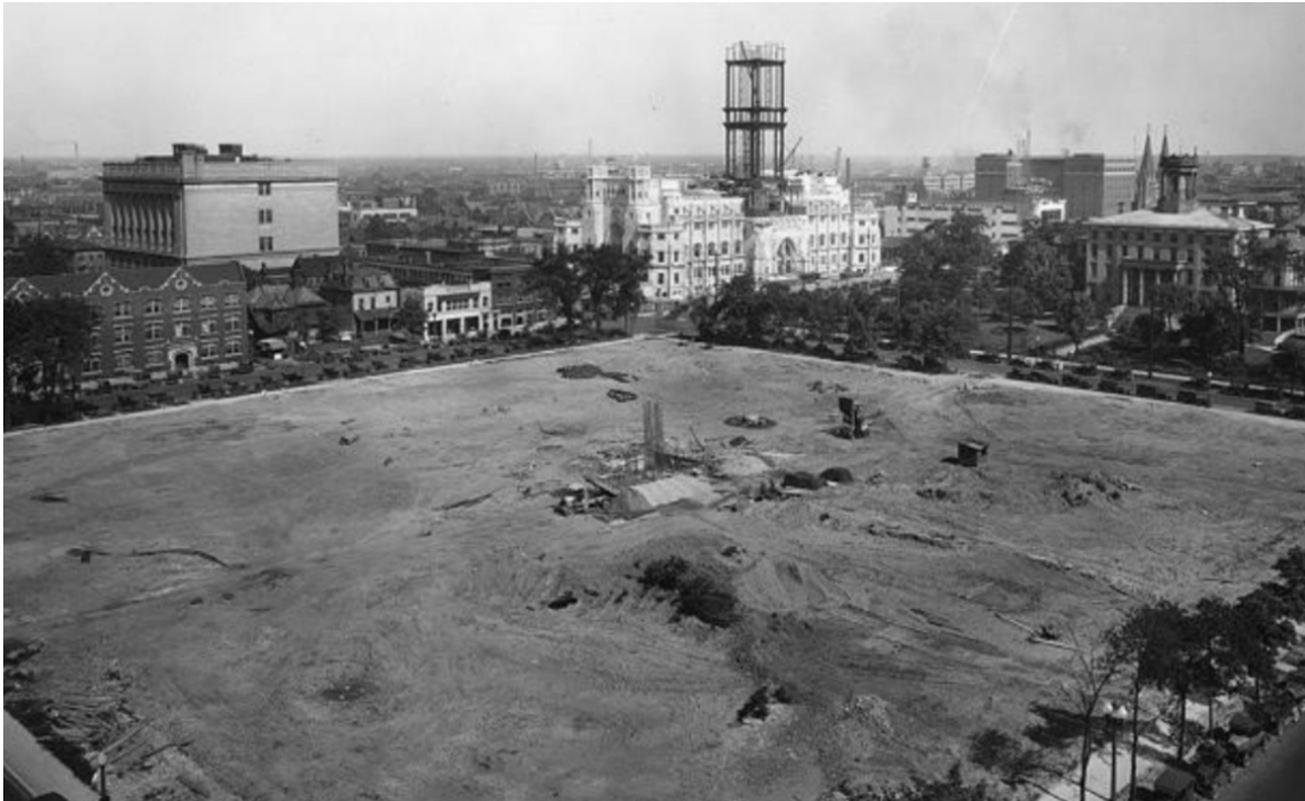
Grading cleared site for Obelisk Square. Between Michigan and North Streets, July 1928. War Memorials Commission
