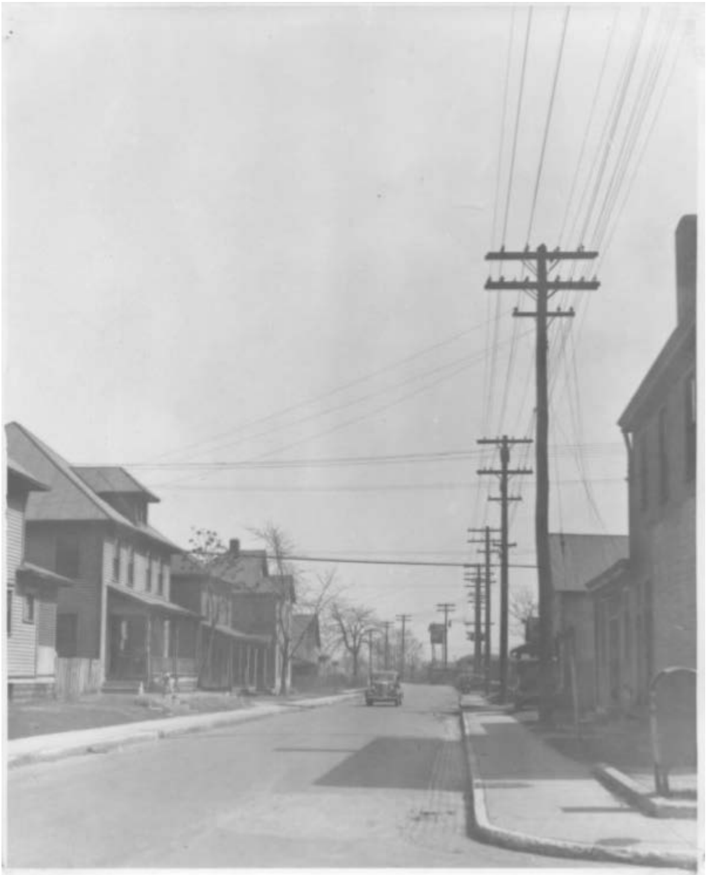
Source: DeeDee Davis, Indianapolis Power & Light Co. Distribution System Photographs Collection.
