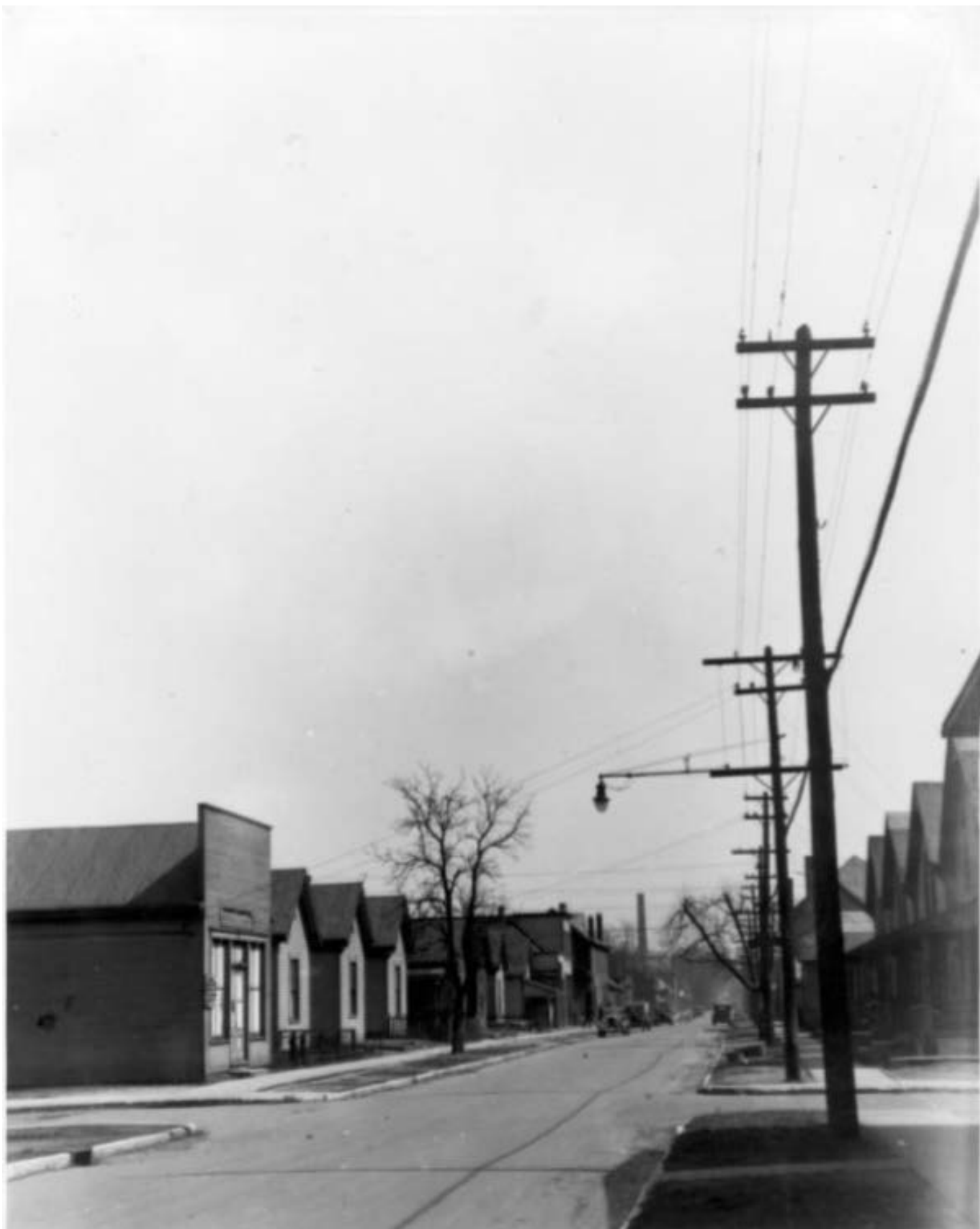
Source: DeeDee Davis, Indianapolis Power & Light Co. Distribution System Photographs Collection.
